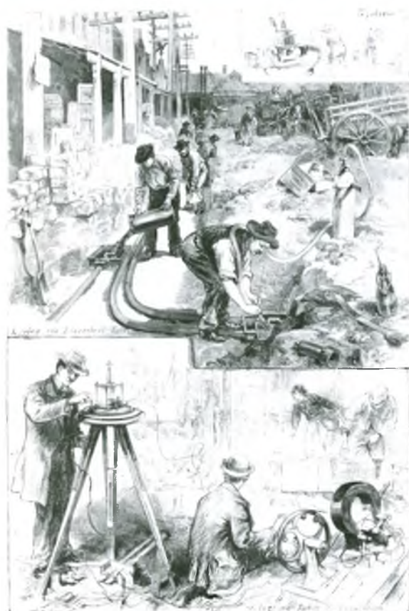
"The electric light in houses—laying the tubes for wires in the streets of New York." Harper's Weekly, June 24, 1882
